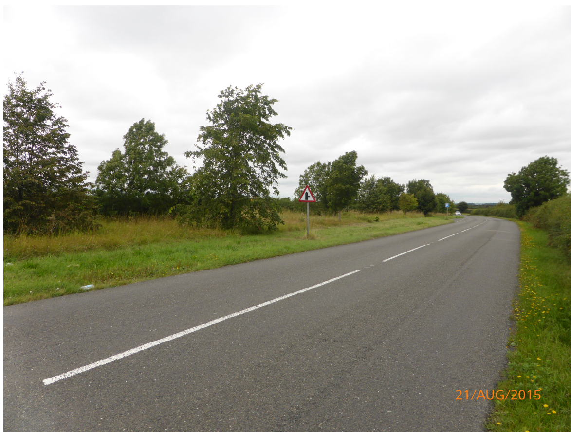
Figure 2.2 The A634 forming the eastern boundary of the site
