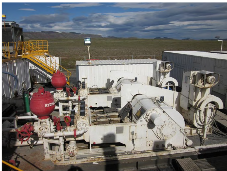
Figure 3.3 Drilling Mud Pumps
