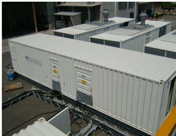
Figure 3.2 Containerised Generators
